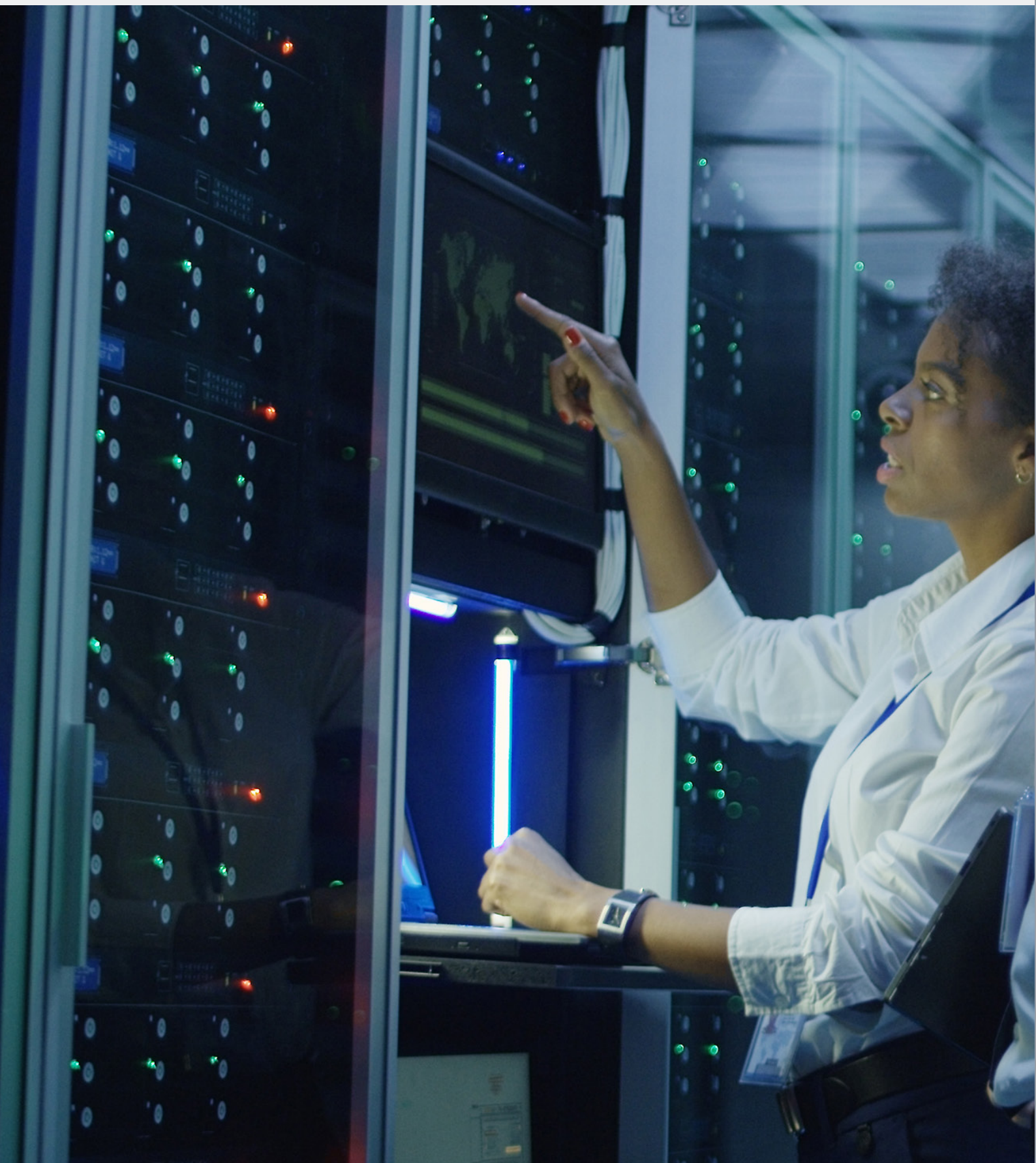
Server room of modern data center. (Photo by FrameStockFootages / Shutterstock.com).
